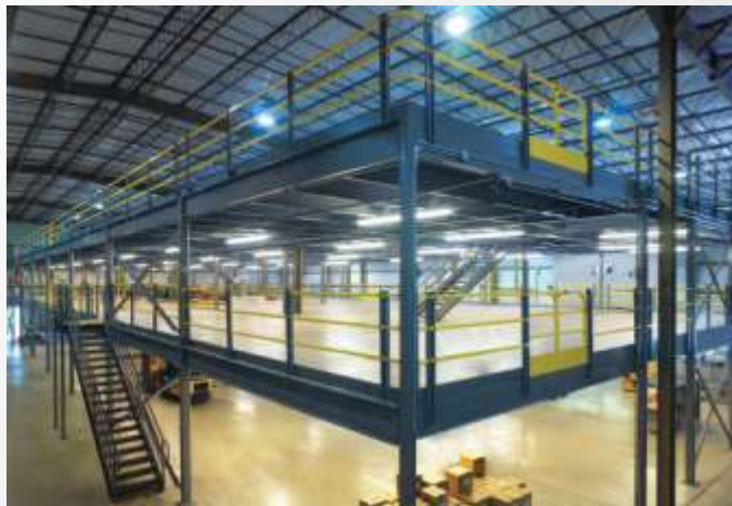
Multilevel Structural Steel Mezzanine
